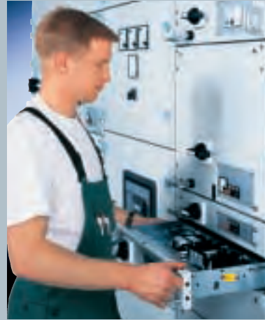
Rapid replacement of withdrawable-unit compartments
